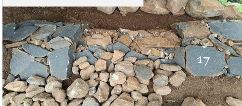
Stone Outlets Created
